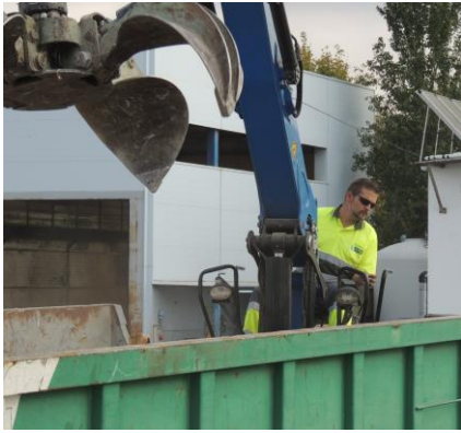
Worker operating a grab crane truck
