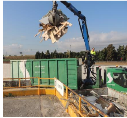
Loading wood on a truck using a grab crane
