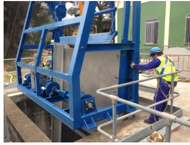
Final phase of the grille installation
