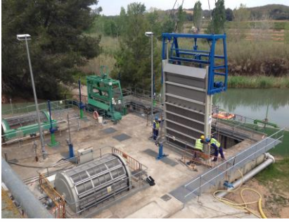
Overview of the intake with new filter and new grille
