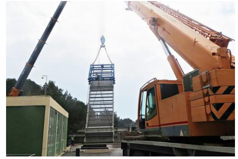
Commencement of the grille installation with two cranes
