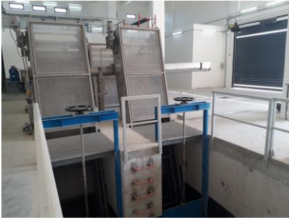
Automatic screens and intake gates.
