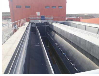
View of the longitudinal bridge for degreasing and grit removal.
