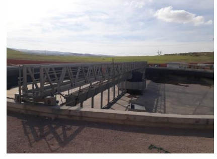
View of a secondary clarifier.
