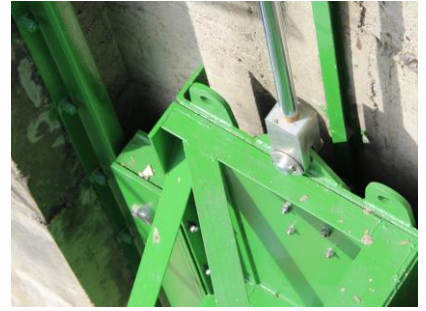
Detail of the sluice hoist system
