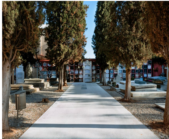
Naturasfalt paving with the polished Boulevard finish and improving flowerbeds and area of graves and mausoleums.
