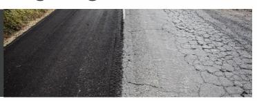
**In-place surface rehabilitation.** This technique permits structural rehabilitation of old surfaces using a homogeneous mixture of milled material from the existing surface, bitumen emulsion, water and possibly additives. All this is carried out at ambient temperature in a single, in-place process.
