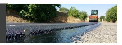
**Elastam is a bitumen emulsion** made from a highly modified bitumen. It is specially designed so that breaking, the residual bitumen is incorporated into the bitumen mix. Adding modified bitumen improves the properties of the final bitumen mix.
