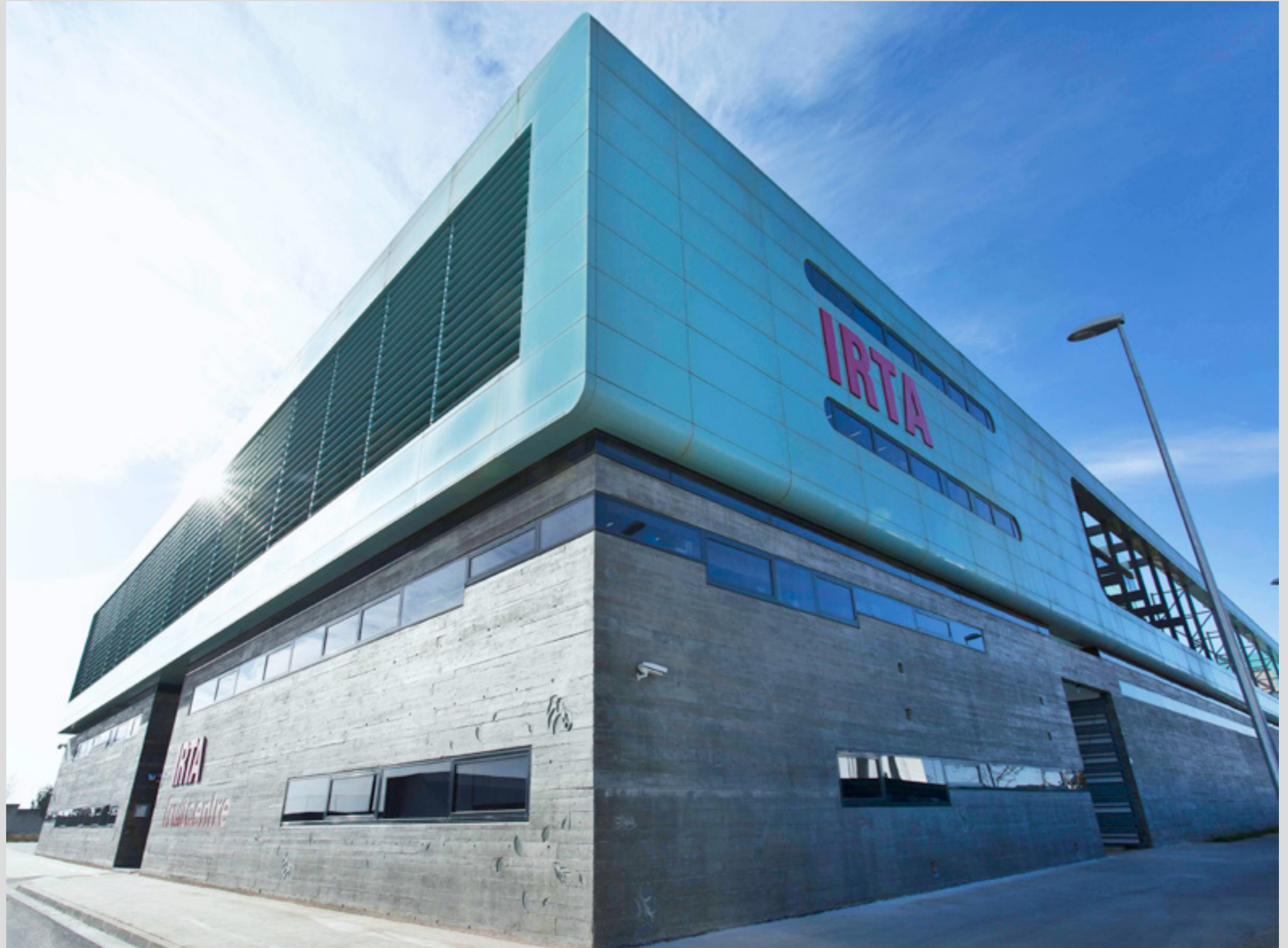
Construction of the Fruitcentre building at the Agri-food Research and Technology Park of Gardeny (PCiTAL), Lleida. PHOTO: Sònia Tapiolas.
