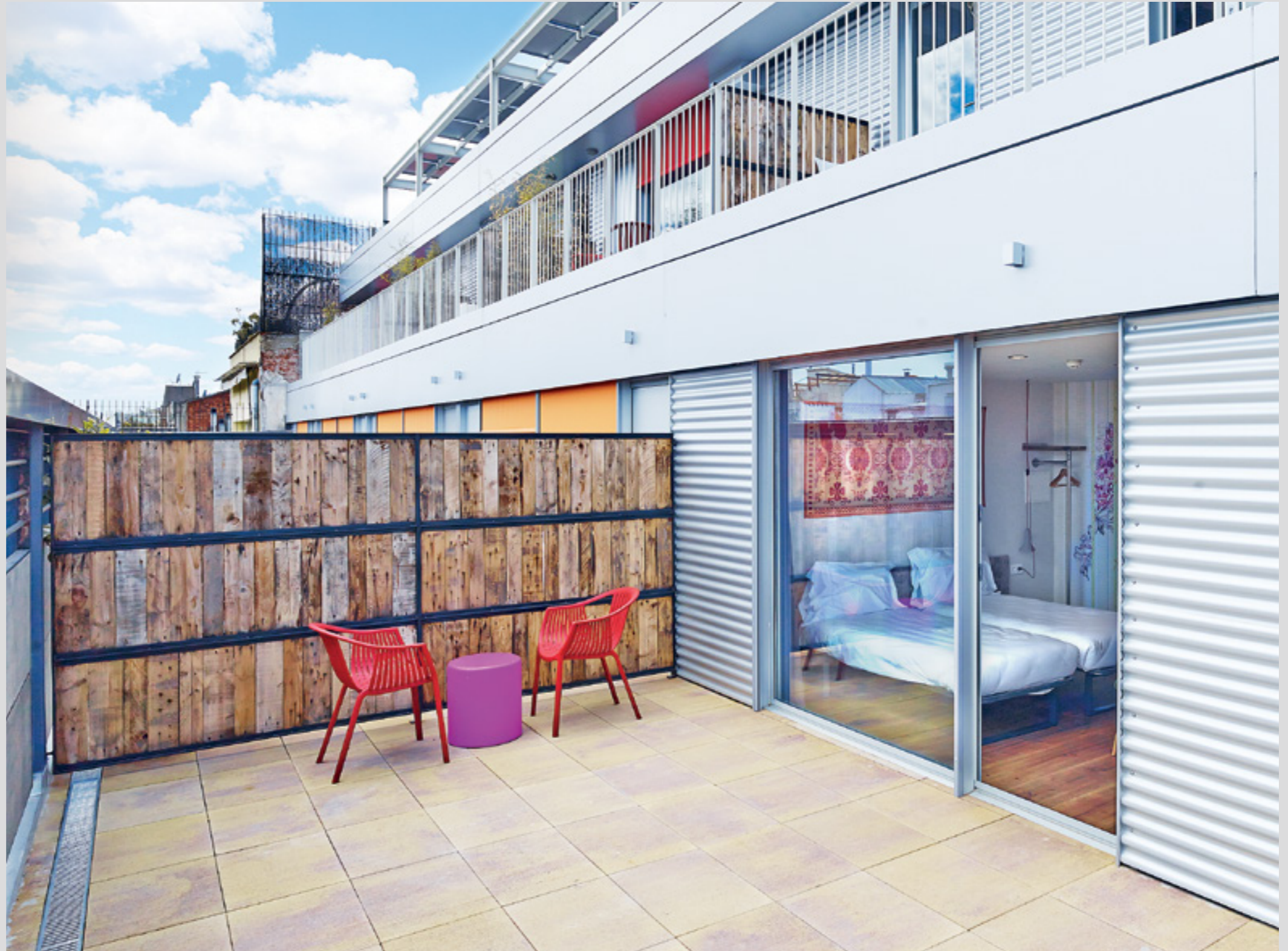
Rehabilitation of a building for hotel use: Generator Hostel, Barcelona. PHOTO: Jordi Bernadó.
