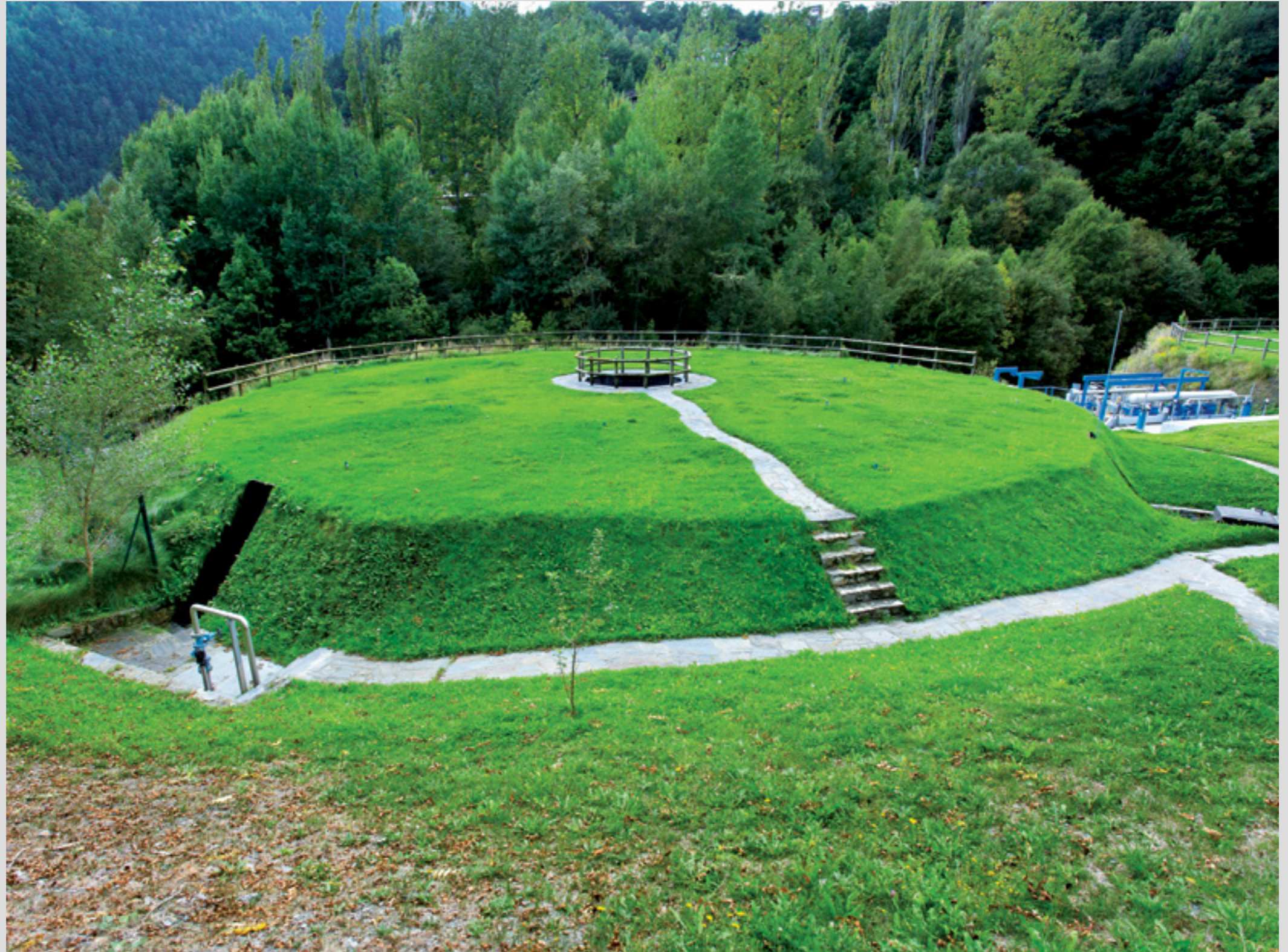
Expansion and improvement of the Northwest WWTP in Andorra. PHOTO: Sònia Tapiolas.
