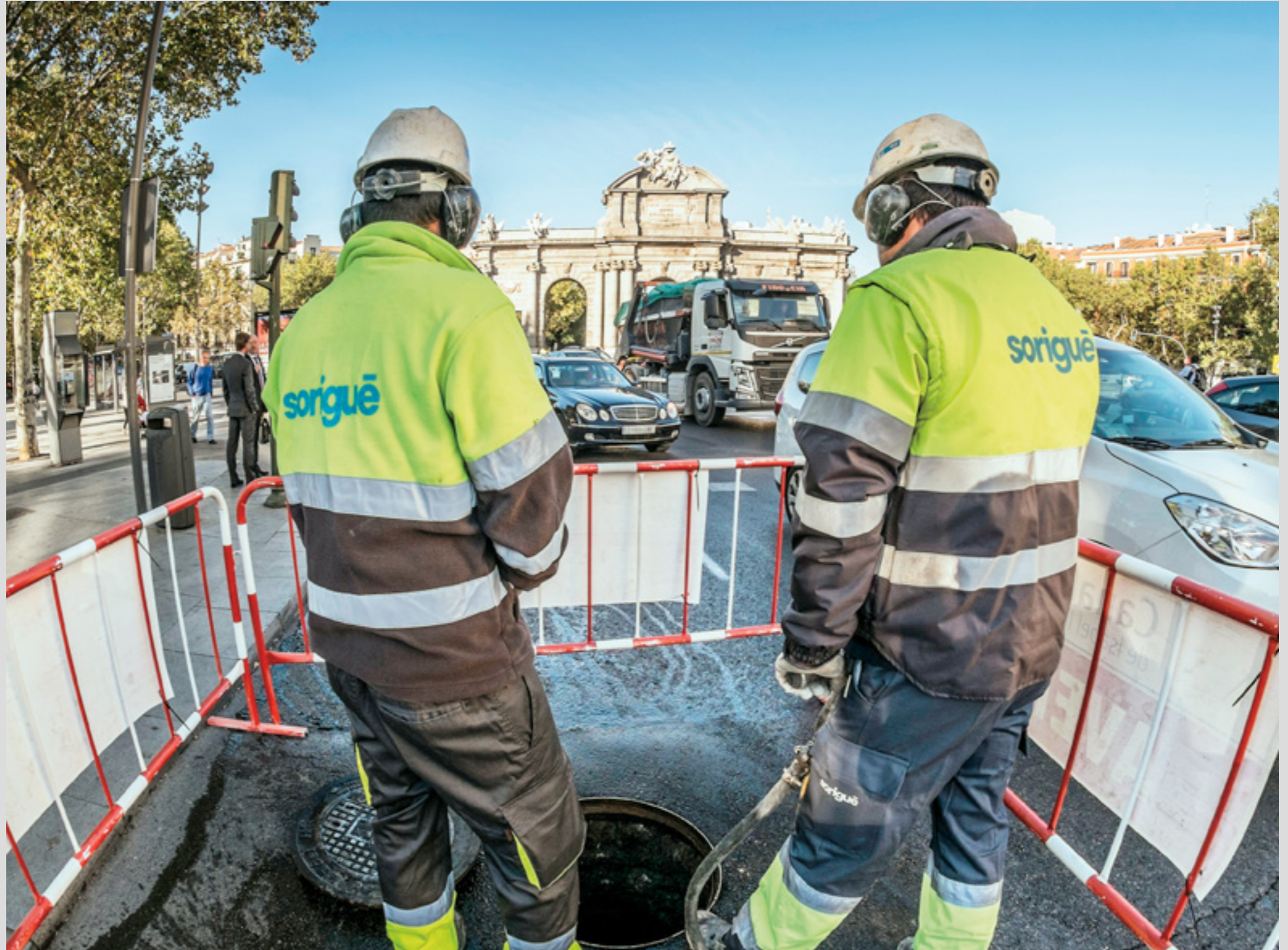
Service for refurbishment and repairs on the Canal de Isabel II supply and reuse network, Madrid
