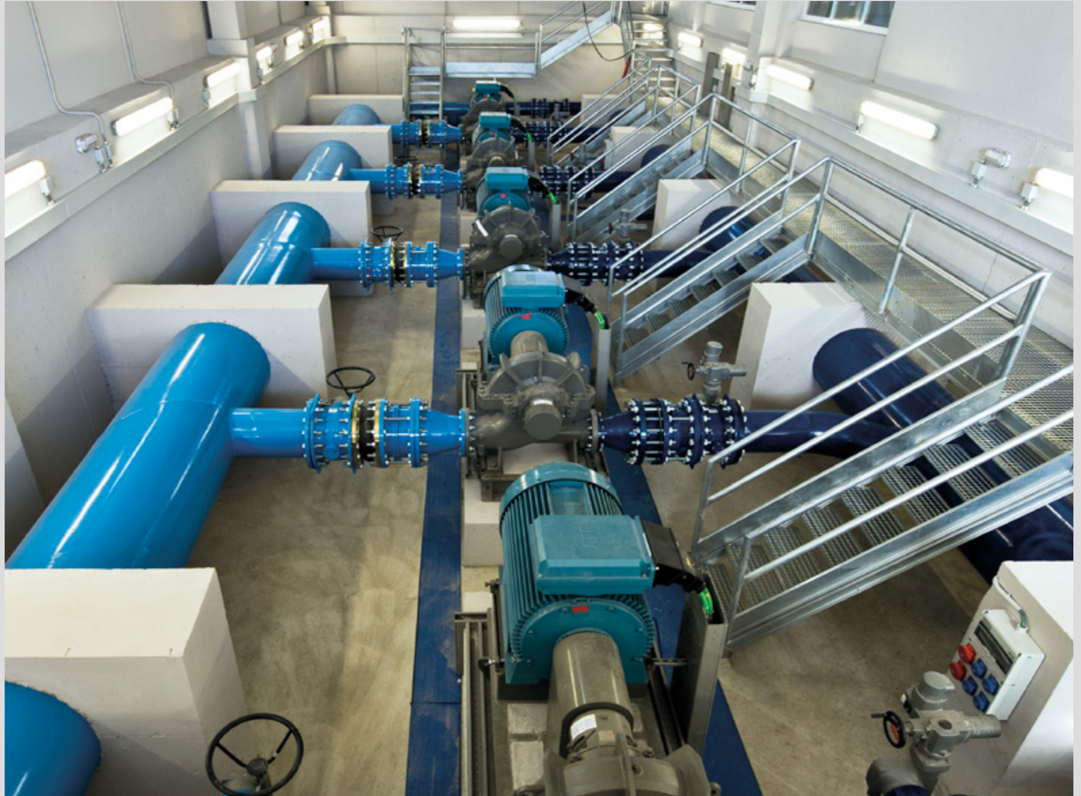
Repair service for breakdowns for the Canal de Isabel II (Madrid) network. PHOTO: Javier Sánchez.
