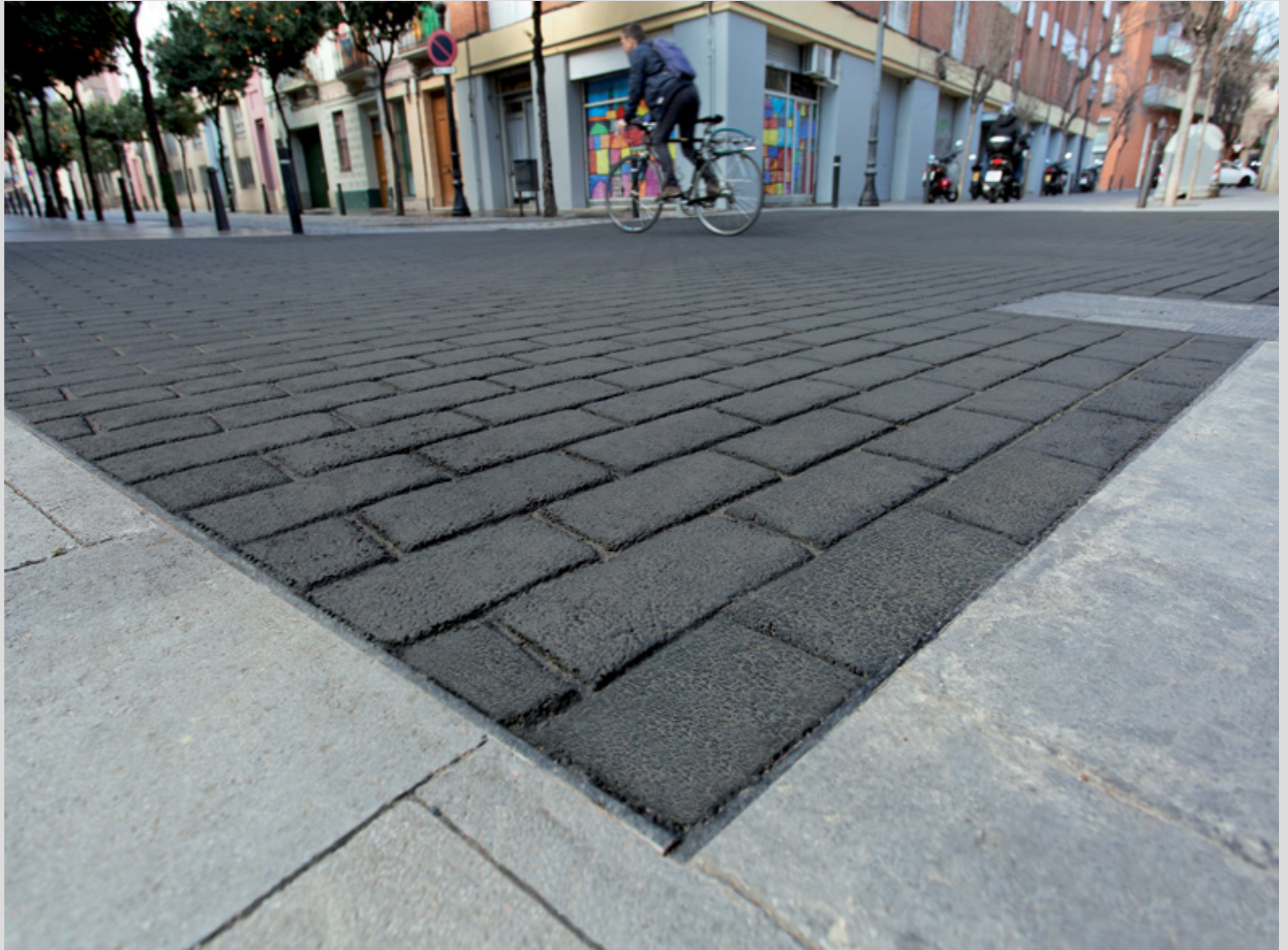
Printed asphalt application, junction in the Sant Andreu neighbourhood, Barcelona. PHOTO: Sònia Tapiolas.
